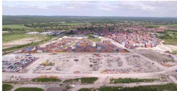
Over 379 timber frames now stand on the Larkhill site, with 283 brick wrapped and all 450 plots have the foundations in and are up to ground floor slab, ready for the remaining timber frames to be erected. Internal works continue, with over 182 homes now plastered and to date over 151 properties have undergone second fix. 153 garages have been completed. All SFA sites are proceeding to schedule. The first handovers are planned for July
